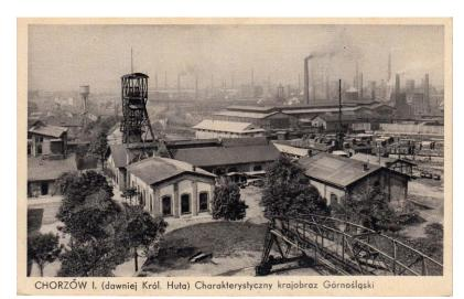
The "Prezydent" (President) Shaft was designed by an engineer Richard Heileman in 1931. His project included: the Shaft Tower, the building of the hoisting machine and the building where coal was sorted. These objects were built in 1933. The Tower had been reinforced by a concrete structure, which distinguishes it from other shaft towers in Europe.
